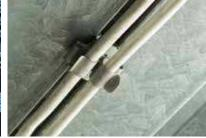
Cable/conduit from composite steel/concrete decking
